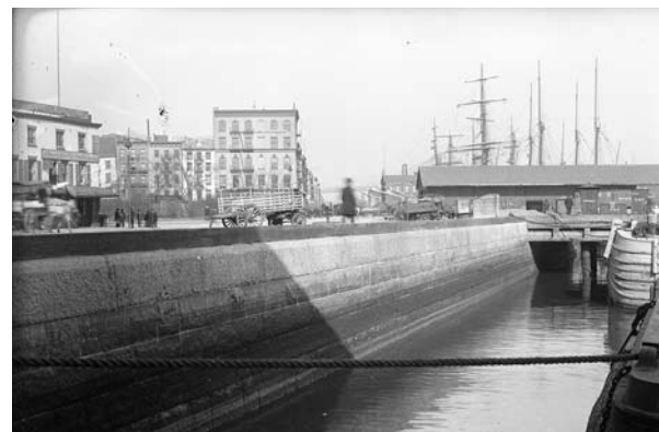
Unlike San Francisco's seawall, New York's riverwall was faced in cut granite blocks. Its vertical face obviated the need for a bulkhead wharf; ships could come right to the wall, which served as the edge of a wharf along the shore. The granite face had a more finished appearance and was more expensive than San Francisco's rubble stone wall.
