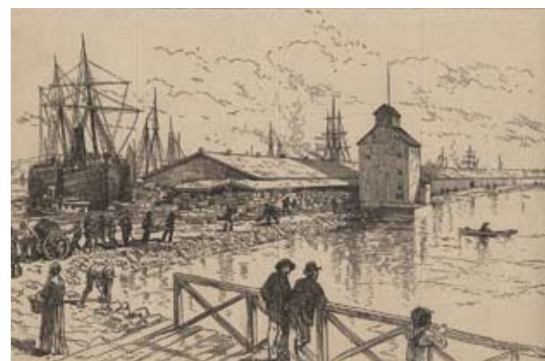
This 1881 drawing from Harper's Weekly shows the gently curving alignment of the redesigned seawall, built from 1878 to 1915 and later extended, before construction of the bulkhead wharf made it possible for ships to unload directly onto the shore.
